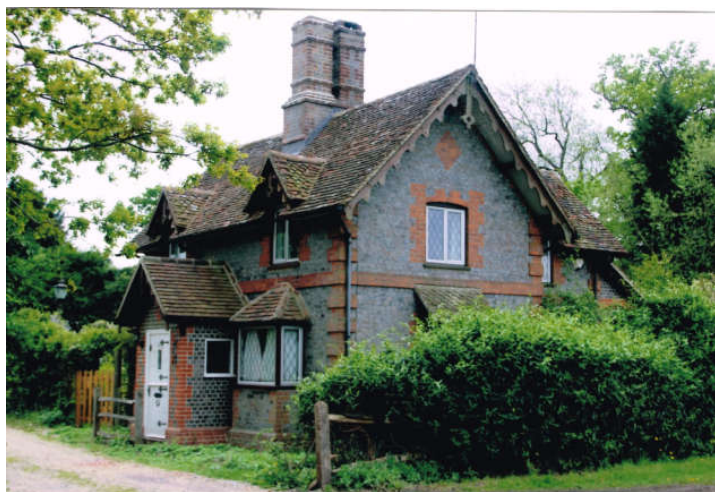
Gate House Plaistow Rd
